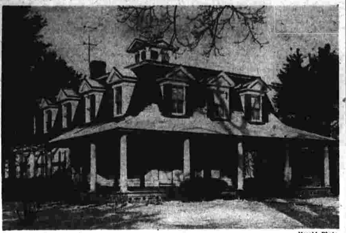
A Christmas wreath hanging on the front door adds a pathetic and tragic note to this scene of the England home at 288 East Center street where four members of that family were wiped out early yesterday in an apparent fratricide murder and suicide. The shootings occurred in a second floor room at the north side of the house. Police today revealed new evidence bolstering their theory that the killings were premeditated and that W. Harry England shot his wife and two children and then killed himself.
